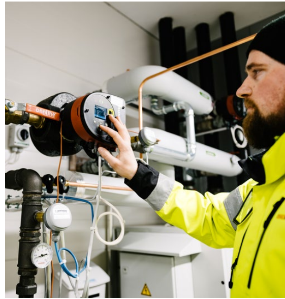
Air-water heating systems and heat pumps for energy-efficiency improving heating renovation projects
